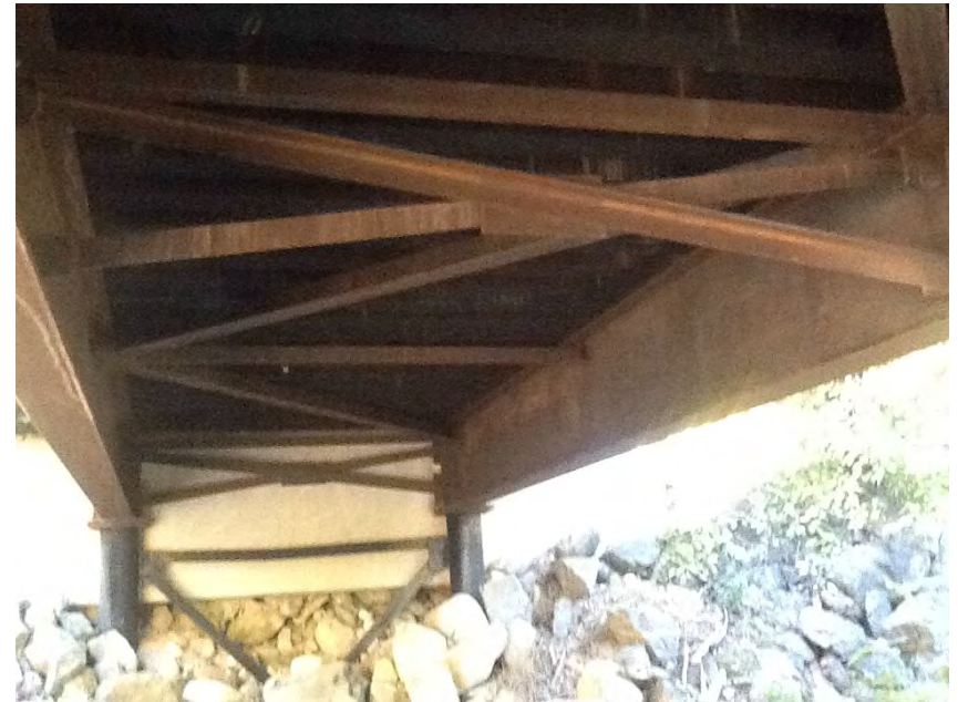
Underside of bridge
