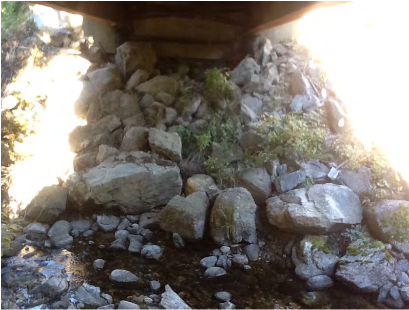
Right Bank Abutment when facing downstream
