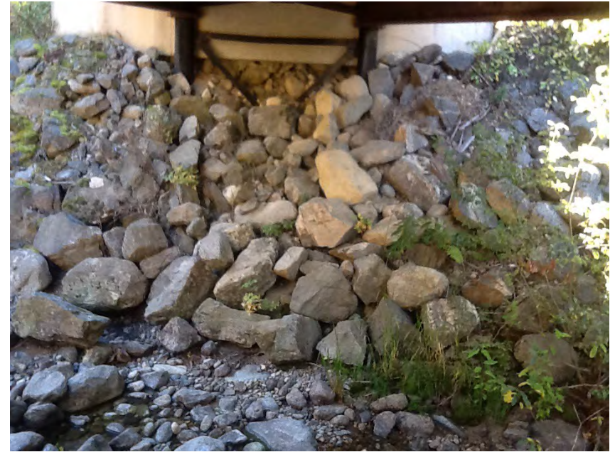
Left Bank Abutment when facing downstream
