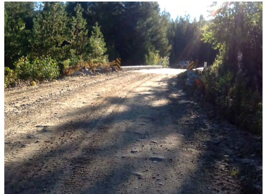
Right approach facing structure
